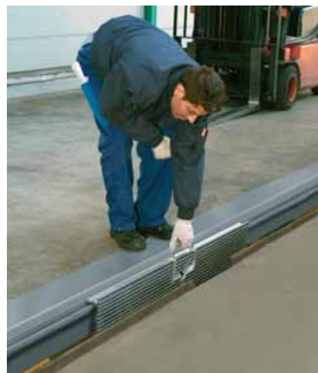
BB bridge lifted out of guide rail.
