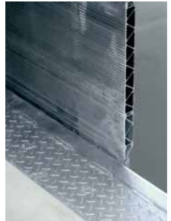
Top plate welded to rail.
