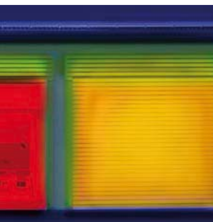
This thermal image of a conventional roller door clearly shows the loss of heat to the outside.
